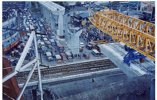
LINE 2 Under Construction
